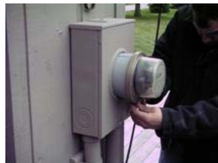
A Power Collar after Installation
